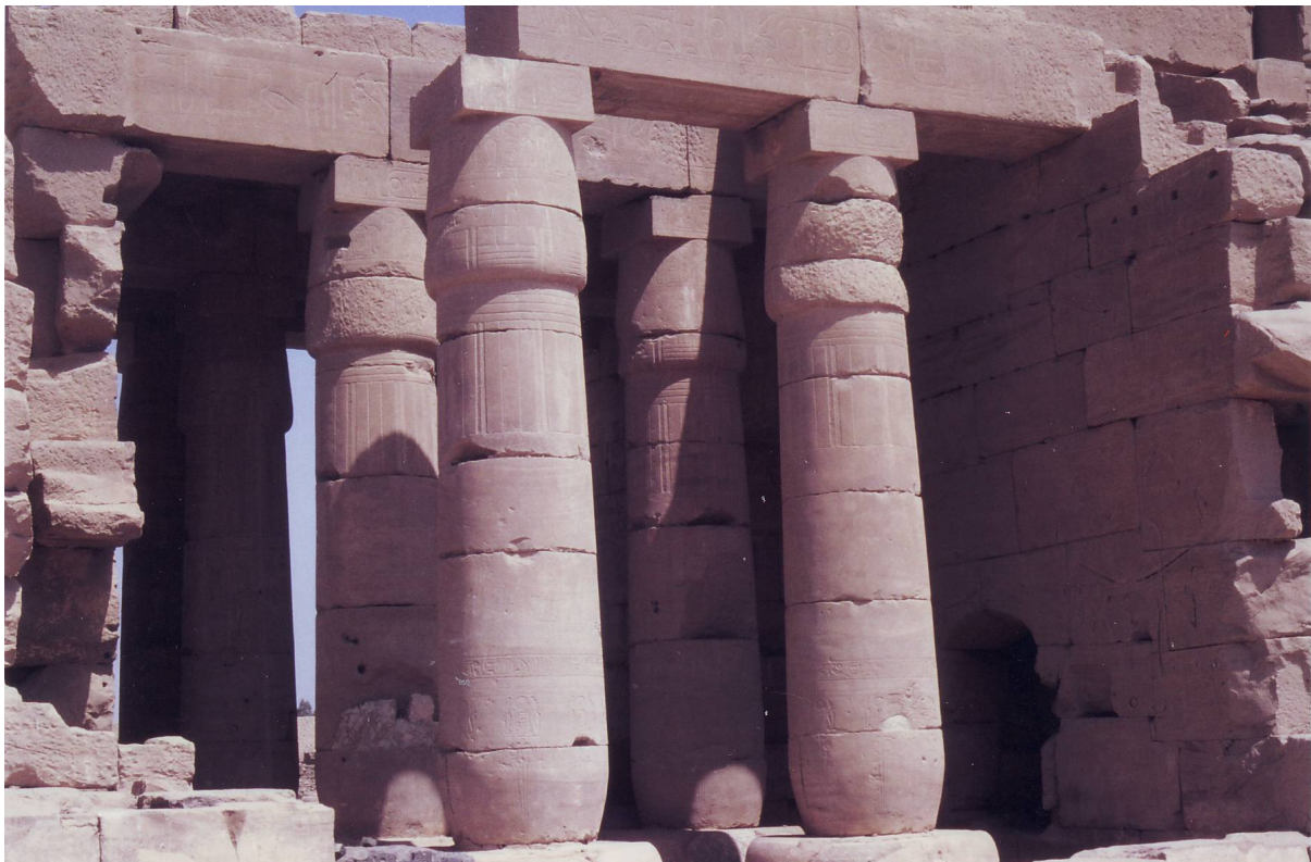
Columns of astronomical room
